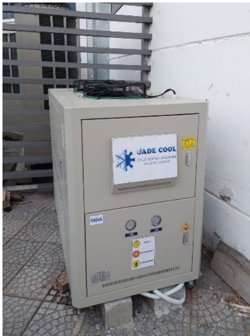
Outdoor unit installed
