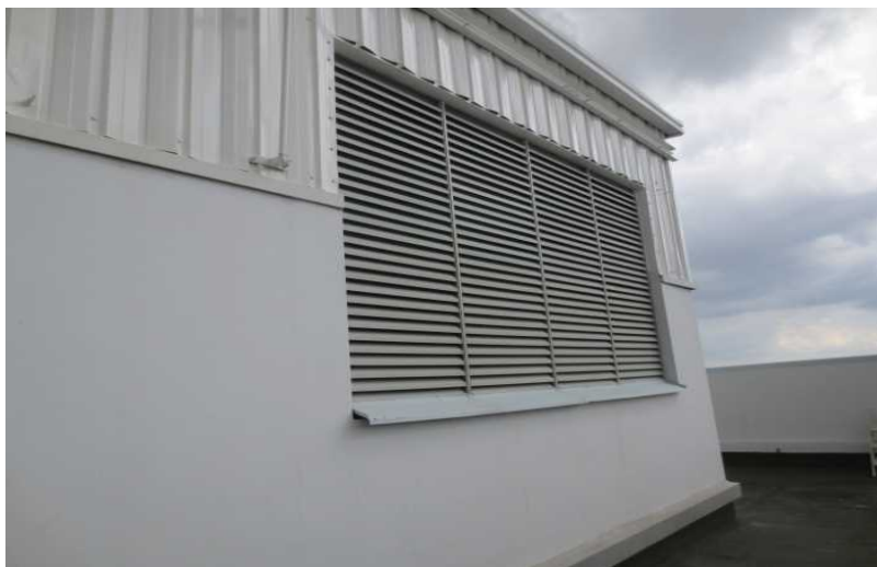
Figure 8 Rooftop Outside Air Intake
