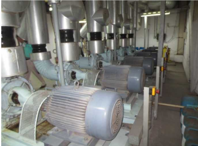
Figure 9 Rooftop Primary Cold Water Pumps
