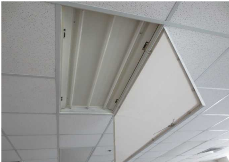
Figure 10 Lighting Equipment (Fluorescent Lights) of a Tenant
