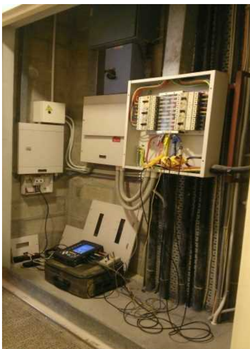
Figure 13 Measurement of Electric Power used in a Tenant Distribution Panel
