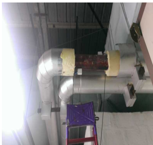
Figure 12 Flow Measurement in Primary Cold Water Pipes on Rooftop
