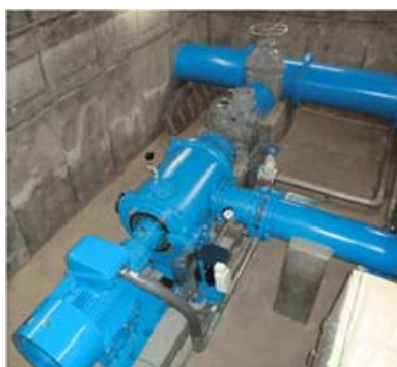
Photo: Linkless Francis Water Turbine Generator
