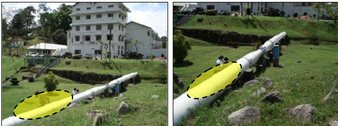
Figure: Expected place to install micro hydropower equipment
