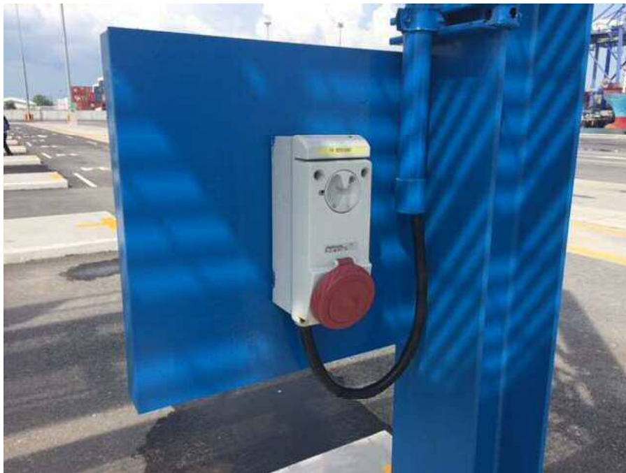
Photo 12: Reefer plug at Coastal-A
