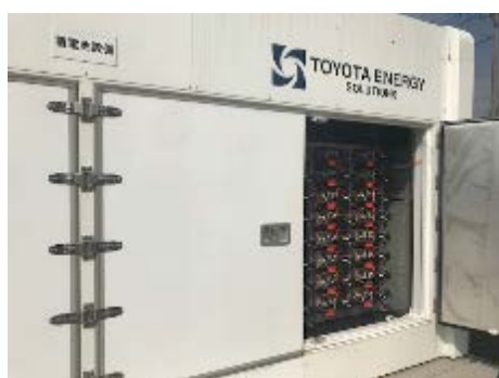
Reuse battery system
