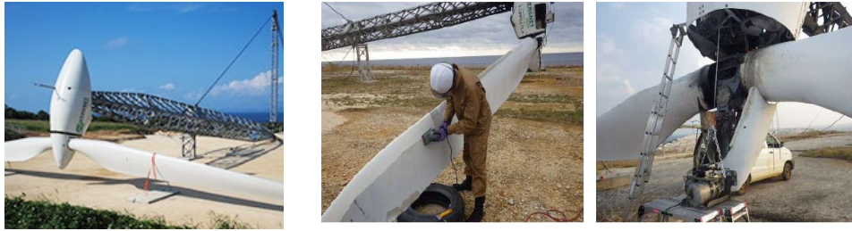
Figure 2-6 Tiltable Wind Power Generator and Maintenance Work after Tilting
