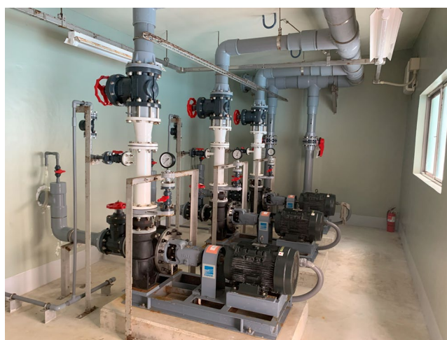
Figure 2-48 Water Intake Pump in the Center
