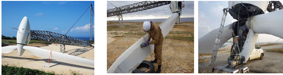
Figure 13: Tiltable Wind Power Generator and Tilting Maintenance
