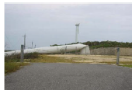
Tower buckled due to typhoon
