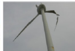
Blade broken by typhoon
