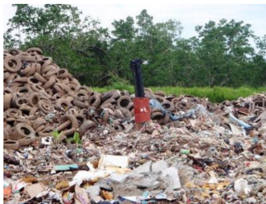
Picture 1.2.1.2 Vent pipe in the Fukuoka method landfill of M-dock
