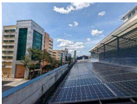
Figure 5-4 On-site photovoltaics in Quezon City Hall
