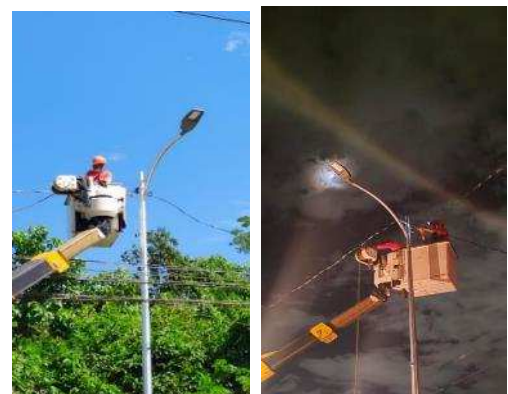
Figure 3-3 Work in progress by Mserv
