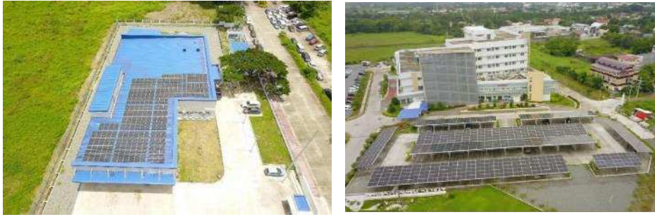
Figure 3-6 BioTechJP's rooftop solar power generation system (left) and Tarlac Hospital's solar carport (right)
