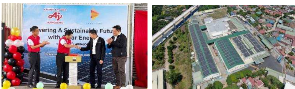
Figure 3-8 1MW solar power generation facility installed in Ajinomoto Philippines Flavor Food Inc.
