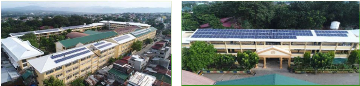
Figure 4-10 Schools with Solar Power Generation Facilities
