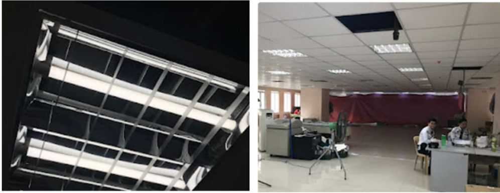
Figure 4-19 Fluorescent Lamps Mainly Used in Quezon City Hall
