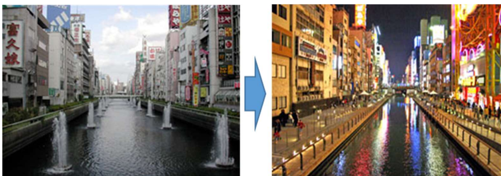
Figure 4-7 Before and After Construction of Tombori River Walk
