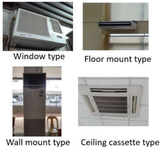
Figure 1-6 Air Conditioners in Quezon City Hall
