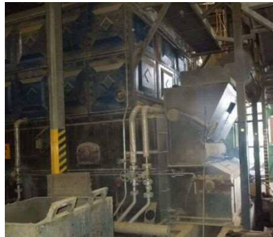
Figure 20: Appearance of 10t boiler
