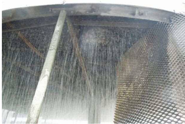
Figure 24: Spraying Condition of the Cooling Tower
