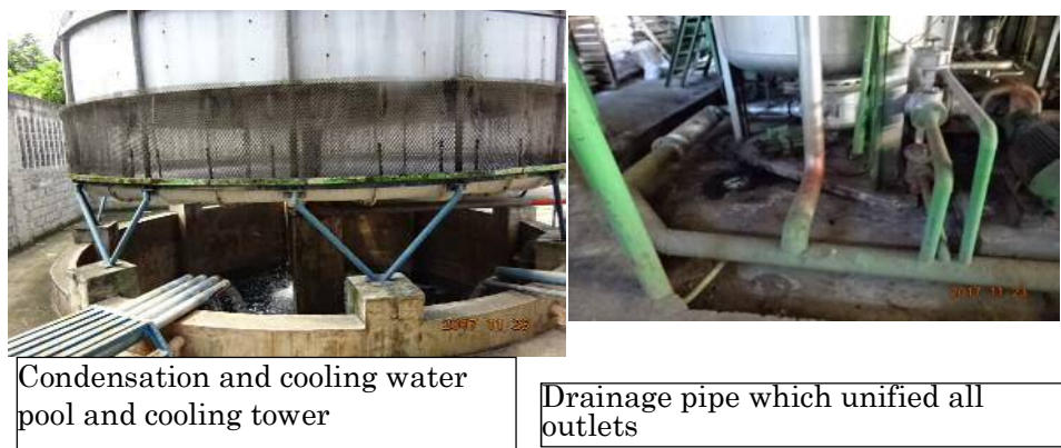
Figure 17: Cooling tower condition
