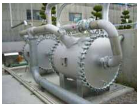
Figure 22: 1-HK type heat exchanger
