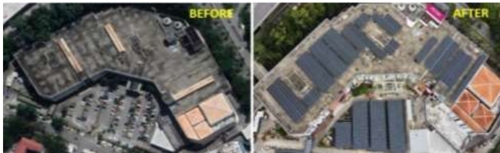
Figure 5.6.1: Aeon's Alpha Angle shopping mall (right: after installation of solar panels) 6
