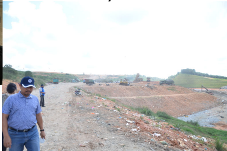
▼ Visit to Seelong sanitary landfill site
