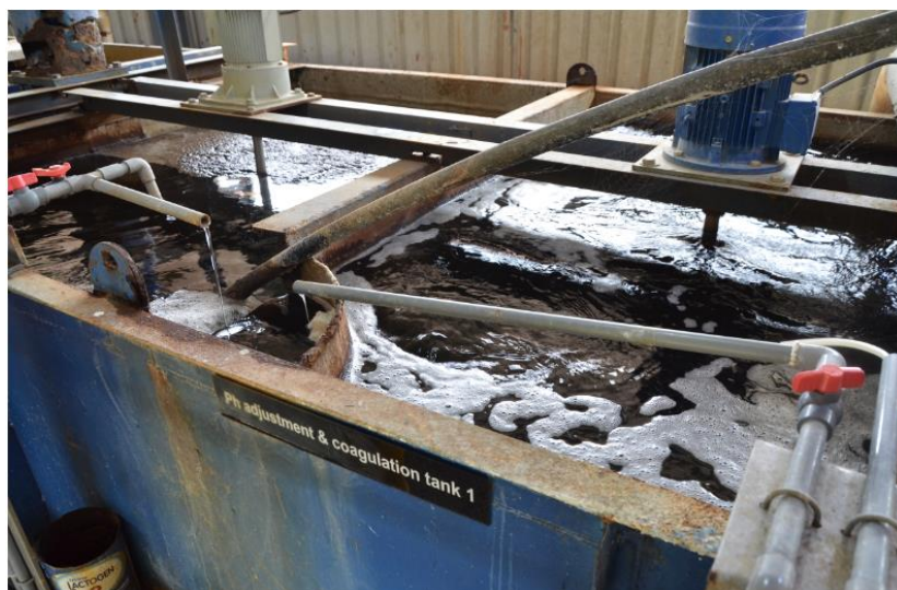
Picture 4-15 (4) Heavy metal removal by Chemical Treatment (Lamellar separator)
