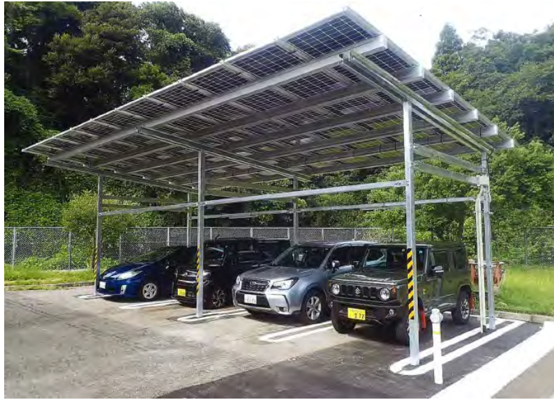
Figure 4-26: Car-port-type solar power system
