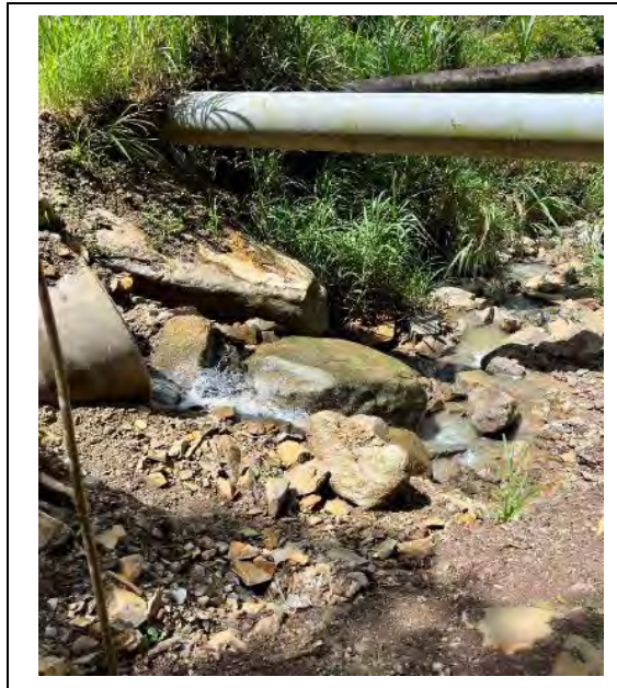
Figure 4-13: Overground penstock from the Mesilou River water intake
