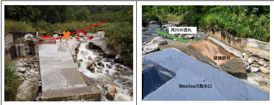
Figure 4-11: Damage caused to the water intake from the Mesilou River
