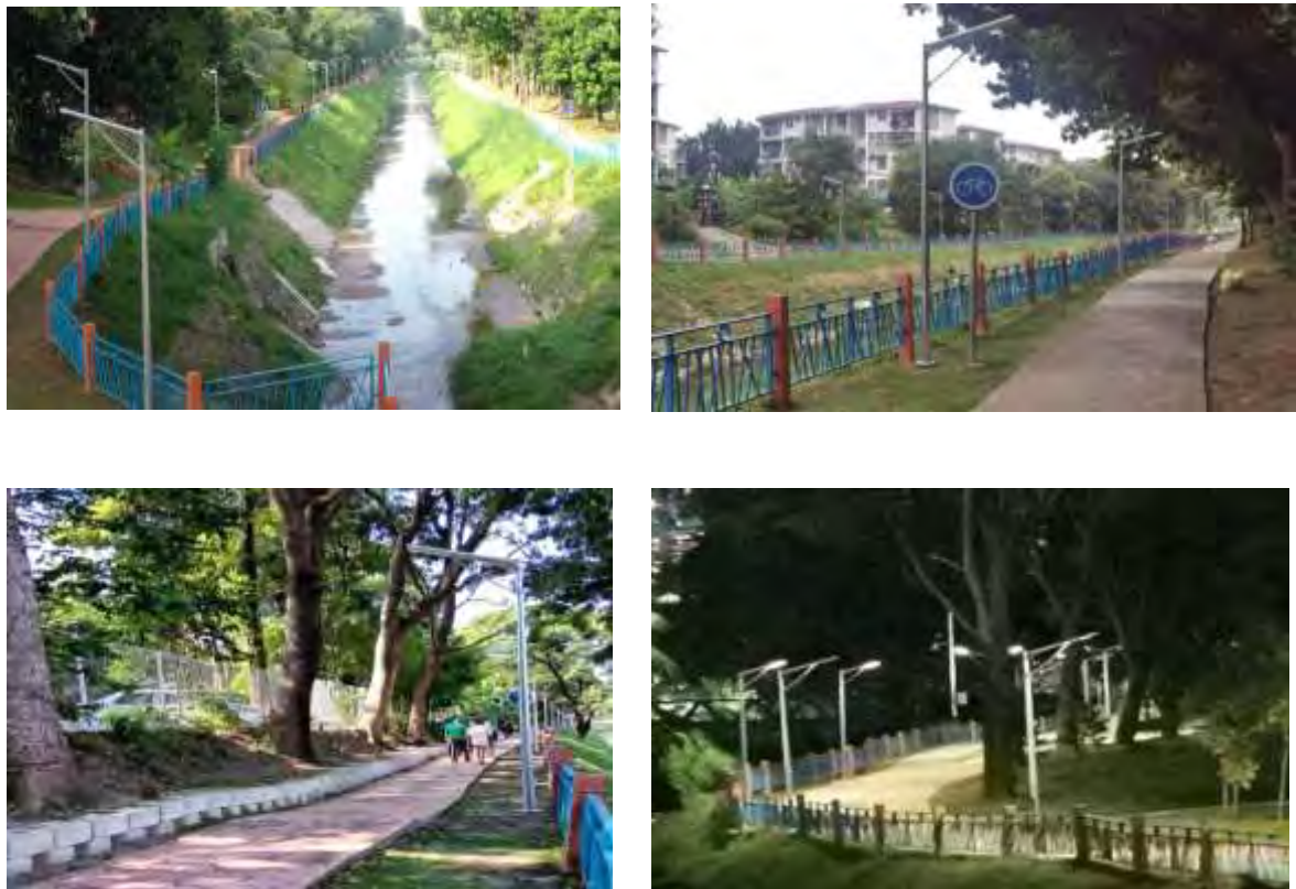
Figure 12: Solar-powered light sticks installed along Bunus River in Wangsa Maju
