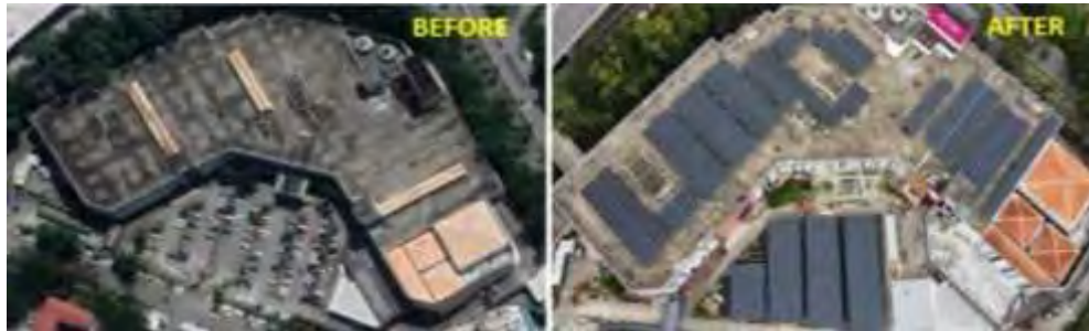
Figure14: Installation of solar panels in the roof and parking area of AEON Alpha Angle Shopping Mall in Wangsa Maju (right figure shows a photo of the mall after solar PV is installed)
