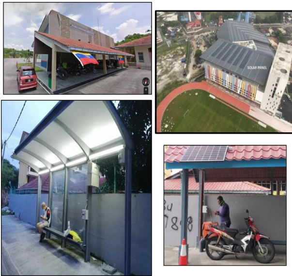
Figure 11: Examples of solar PV installations
