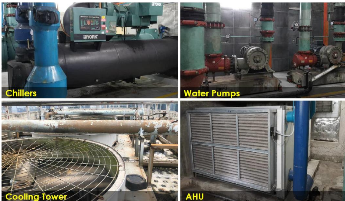
Figure 10: Appliances scheduled to be refurbished
