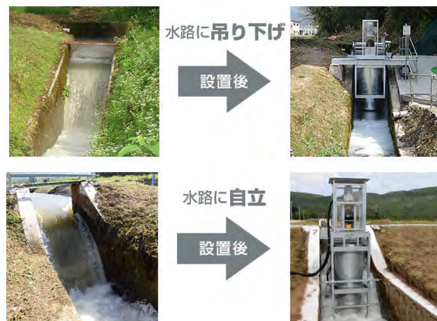
Figure 4-17 Case of installation of Power Archimedes of Hokuriku Seiki Co., Ltd.
