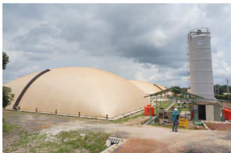
Figure 3-13 Covered lagoon method
