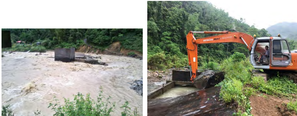
Figure 4-14 Photographs of a river stricken by a flood and staff removing earth and sand
