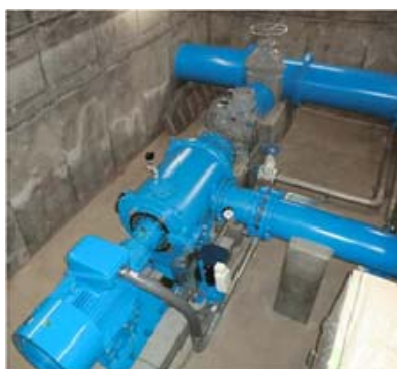
Photo: Linkless Francis Water Turbine Generator
