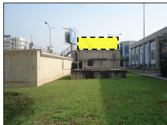
Estimated location to install micro hydropower generator
