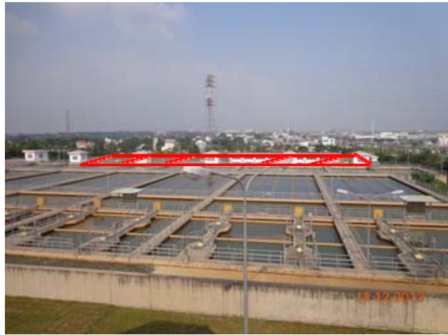
Figure: Estimated place to install the solar power generator
