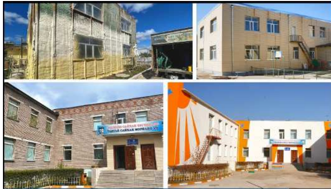
Figure 2-13 Schools refurbished with heat insulation
