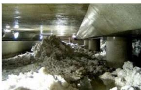
Utilization of cold heat of snow (area around Sapporo Station North Exit) (snow in a melting tank used as a cold water heat source)
