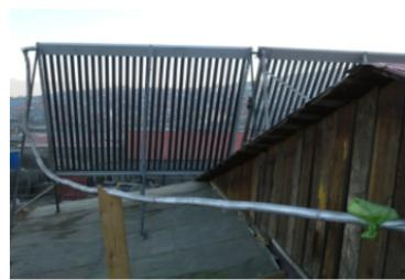
$$\eta_K = \frac{\dot{m} C_p (T_3 - T_4)}{A_c G}$$
