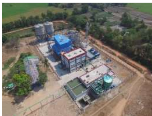
Figure3-1 Outline of rice husk power generation facility in Myaungmya
