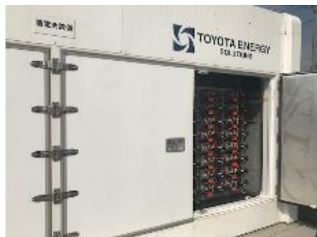
Reuse battery system
