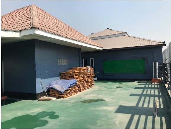
(c) Roof of hotel main building
