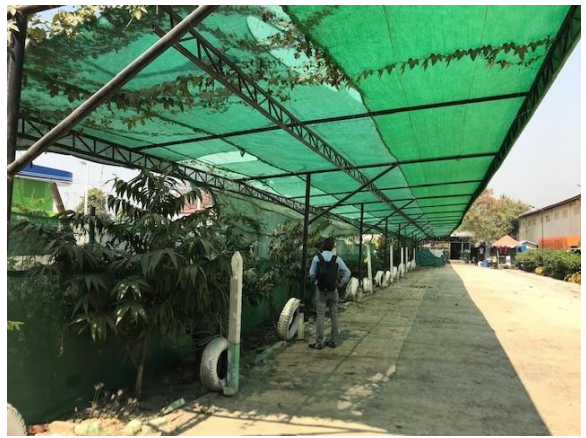
(f) Supporting structure of hotel parking lot
