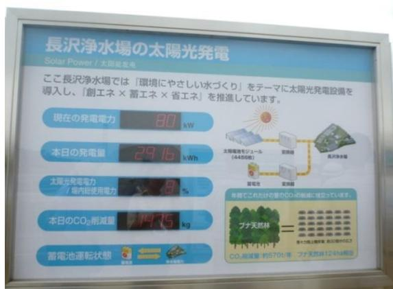
Monitoring panel for showing generated electricity
