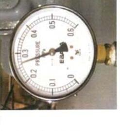
Discharge pressure gauge = 0.26 MPa
