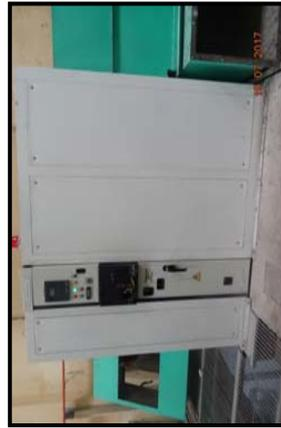
12KV, 1250A Incoming Panels, Bus-Coupler Panel and 630A Feeder Panels of Sub-Station
