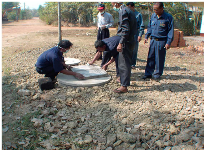
Chart 4-12: Situation of disposal under the ground-2
