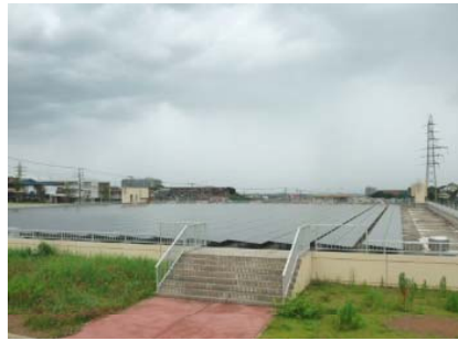
PV modules installed above reservoir
