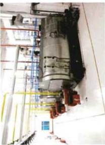
• Gas boiler in oil company office building
