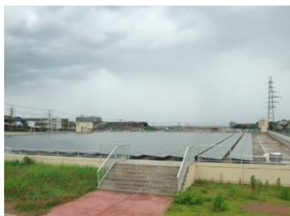
PV modules installed above reservoir
