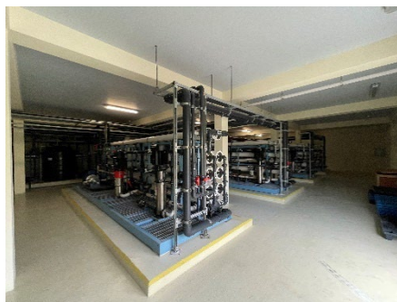
Seawater desalination equipment (RO)
