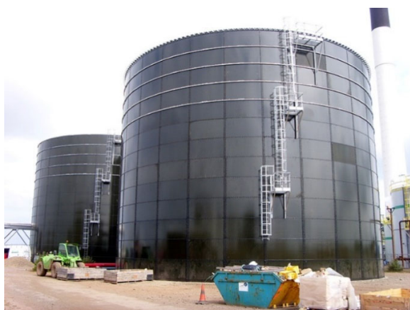
Photo 4.2.1 Methane fermentation tank※
