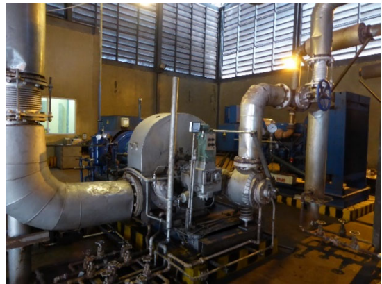
Photo 3.1.5 Turbine/ Generator
