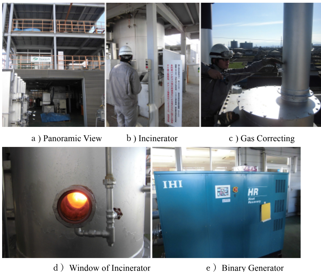
Figure 3-16 : Dry Distiller Gasifier and Binary Generator
