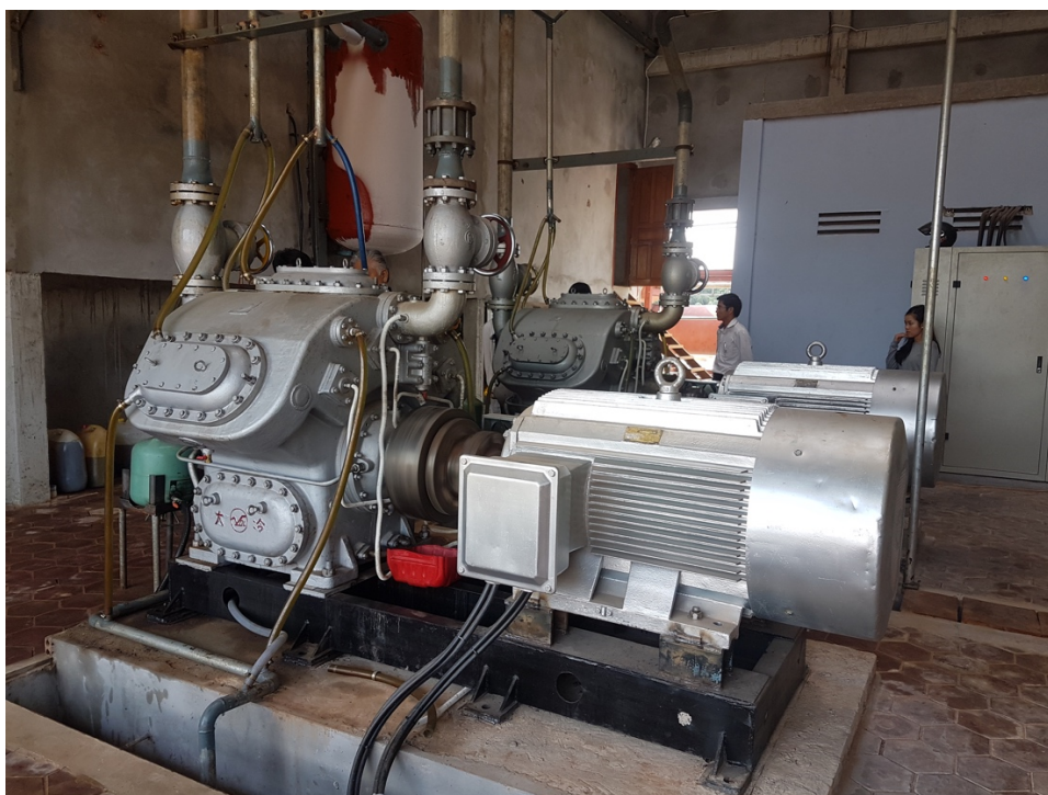
Figure 3-15 : Compressor with the rated power of 150 kW
