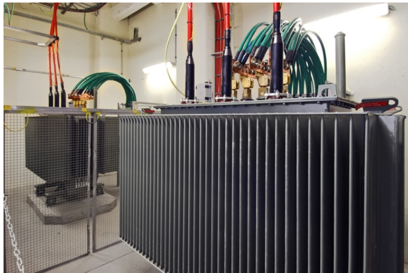
Figure 3-9 : Power from grid step down by Transformer in B-Hotel
