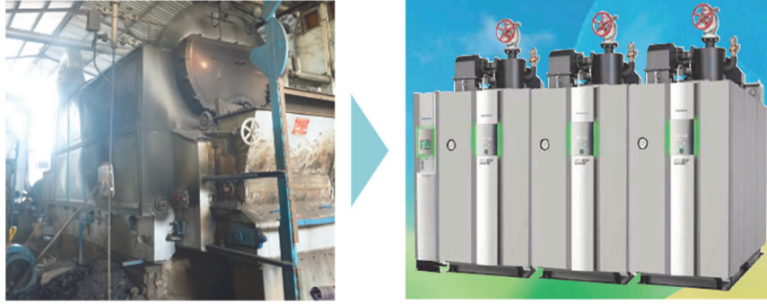
Figure 3.4 Replacement from Coal Boiler to Gas Once-through Boiler
