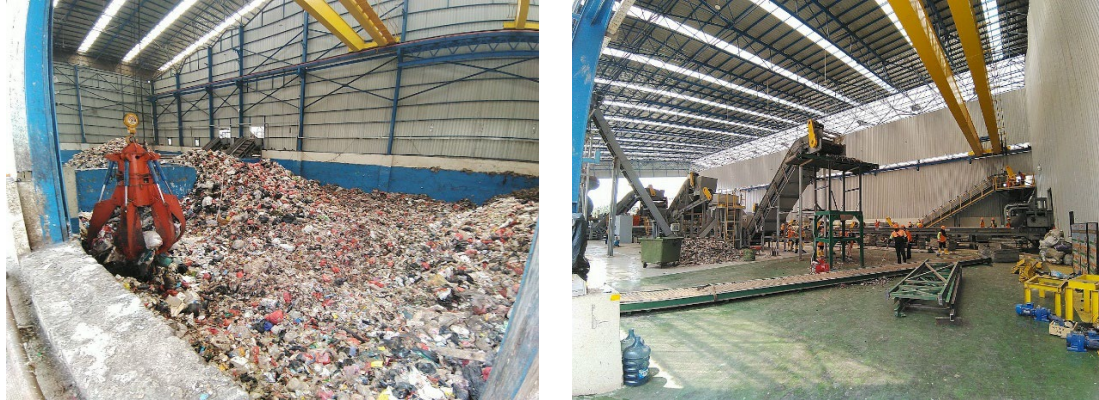
Figure 2.3.1.3.5. Receiving and storage pit for fresh waste (left) and sorting line (right) at TPST Bantar Gebang RDF facility (Source: Photos by survey team)
