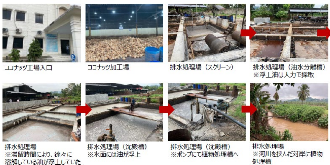
Figure 3-24 Current wastewater treatment flow at PT. Royal COCONUT (created by Aiken Kakoki K.K.)
