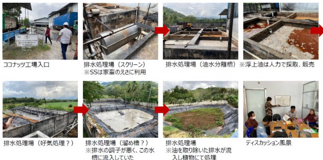
Figure 3-27 Current wastewater treatment flow in PT. Trijaya TANGGUH (created by Aiken Kakoki K.K.)
