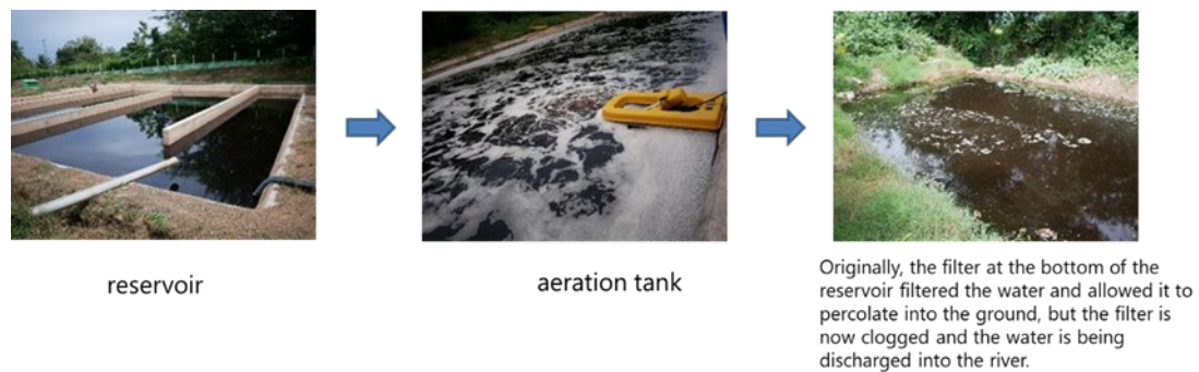
Figure 3-37 Current final disposal site leachate treatment flow
