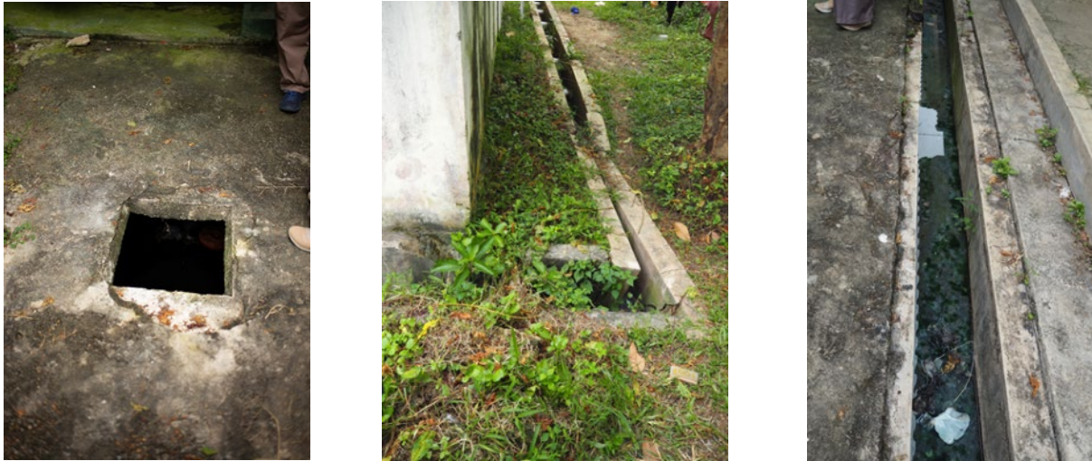
Figure 3-14 Wastewater treatment in the female dormitory (left: human waste treatment (septic tank); right: domestic drainage channel)
