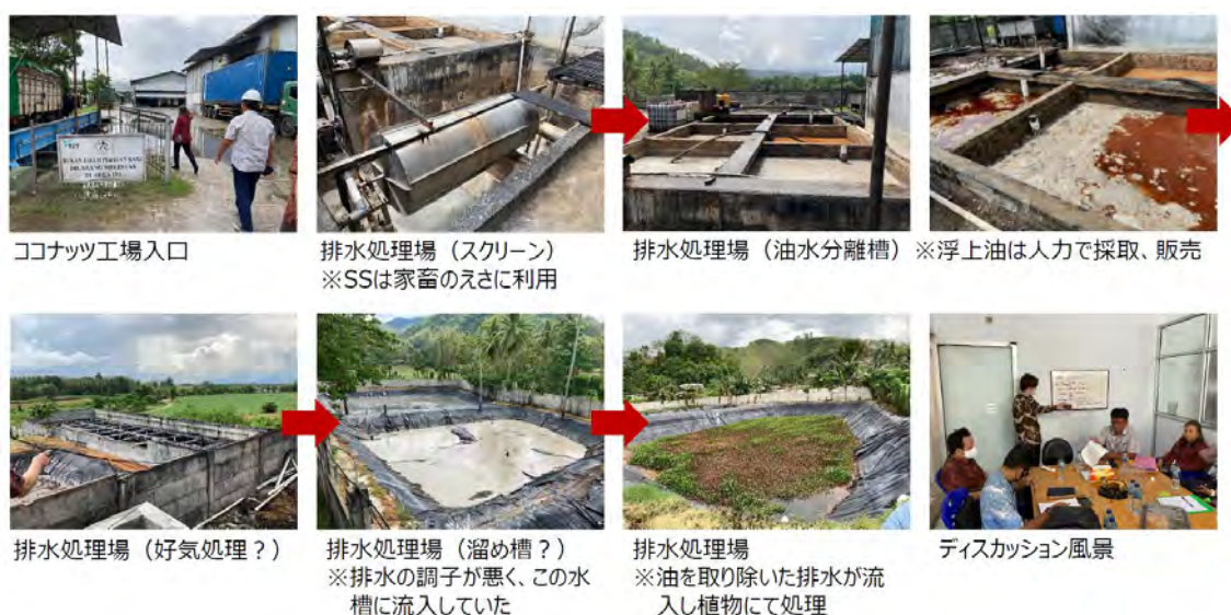
Figure 3-2 2 Current wastewater treatment flow in PT. Trijaya TANGGUH (created by Aiken Kakoki K.K.)
