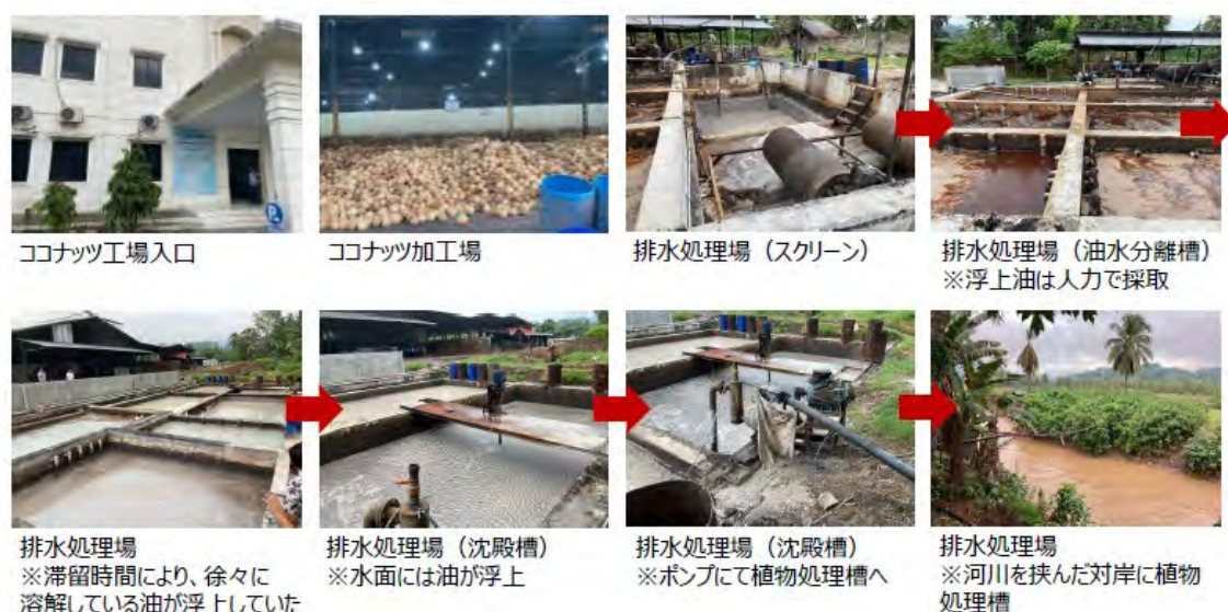
Figure 3- 1 9 Current wastewater treatment flow at PT. Royal COCONUT (created by Aiken Kakoki K.K.)
