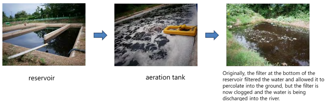
Figure 3-2 8 Current final disposal site leachate treatment flow
