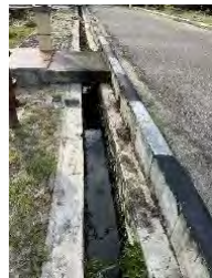
▲ Drainage canal by the building collects wastewater to drainage canal outside the school.
