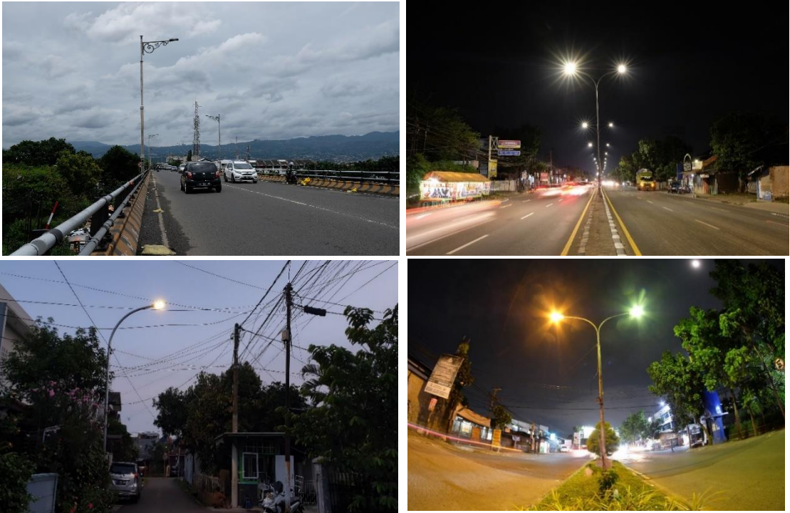
Figure 3-5 On-site inspection (photo)
