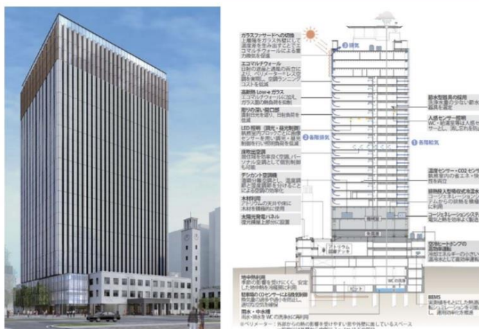
Visualization of New Kawasaki City Hall Building (Left: Entire view of the building; Right: Cross-section of the structure)
