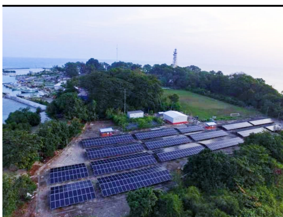
Photo: Solar System on Sebira Island (Photo provided by DKI-JKT)
