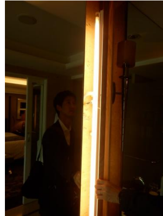
Figure 3-34 Bathroom lighting (indirect) (Fluorescent lamp, inside view)
