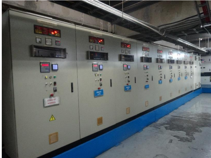
Figure 3-20 Electricity intake equipment
