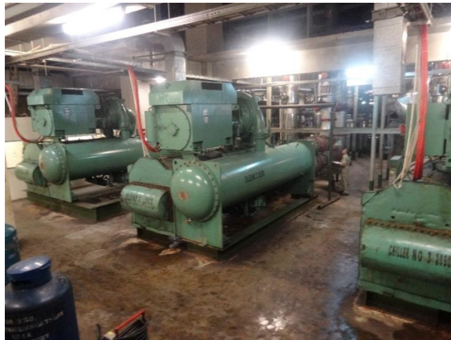
Figure 3-14 Turbo chiller
