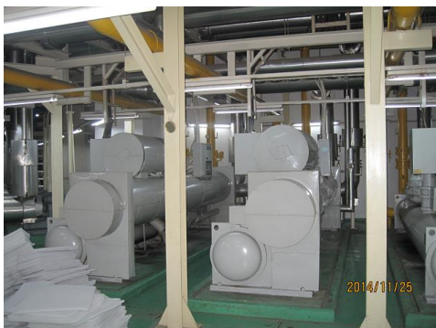
Figure 3-47 Centrifugal chiller
