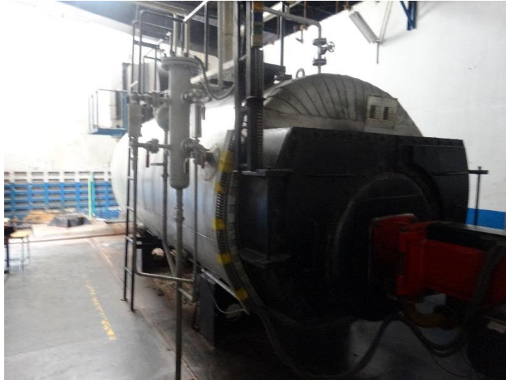
Figure 3-42 Gas boiler
