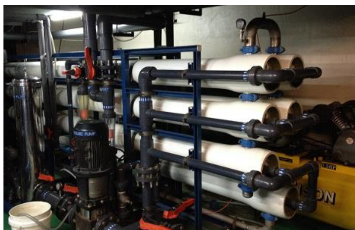
Figure 3-19 RO membrane equipment
