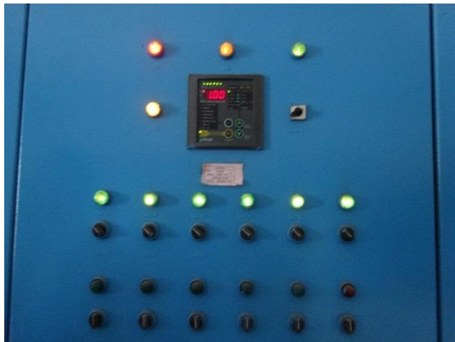
Figure 3-41 Electricity intake equipment panel
