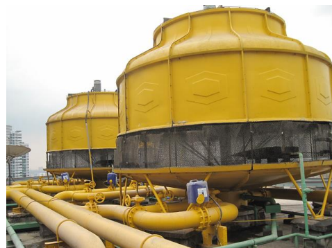
Figure 3-48 Cooling tower
