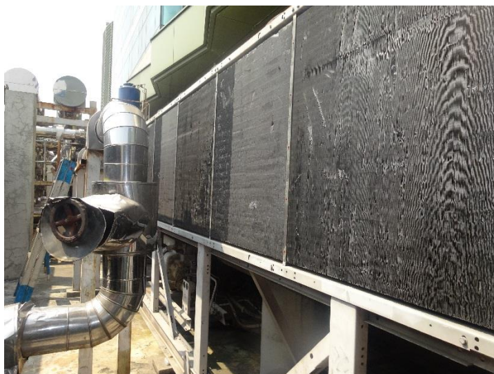
Figure 3-22 Air-cooling chiller
