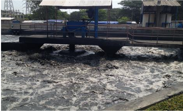
Figure 3-45 Drain treatment tank
