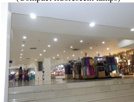
Photos 22: Store passage lighting (Compact fluorescent lamps)
