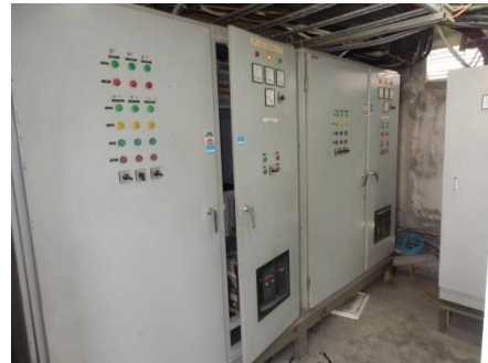
Photo 4: Air-cooled chiller distribution boards (Mall System 2)
