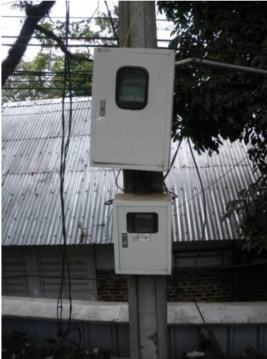
Photo 1: Smart box (top) Power-receiving box (bottom)
