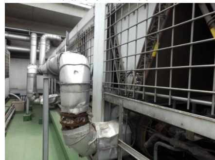
Photo 51: Air-cooled chiller piping
