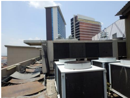
Photo 3: Air-cooled chillers (Mall System 2)
