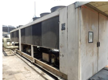
Photo 43: Air-cooled chiller (Mall System 1)
