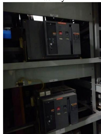
Photo 35: Chiller 1C System breaker (top)
