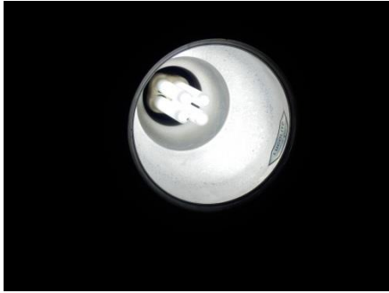
Photo 24: Compact fluorescent lamp (Vertical installation)
