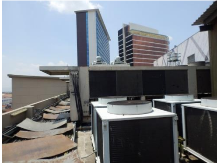
Photo 44: Air-cooled chillers (Mall System 2)
