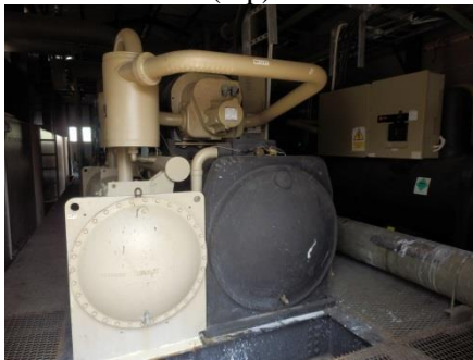
Photo 38: Water-cooled chiller
