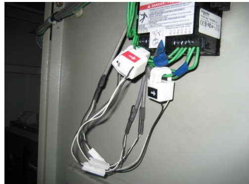
Photo 4: After installation of CT (for chillers)
