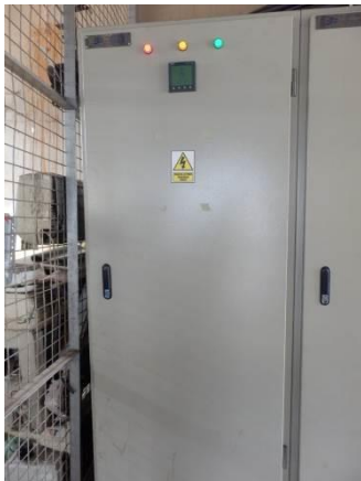
Photo 40: Water-cooled chiller distribution board
