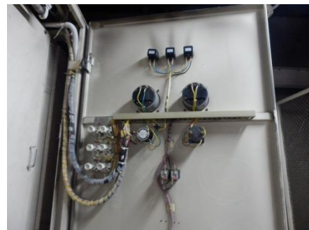
Photo 47: Transformer System No. 2 instruments back
