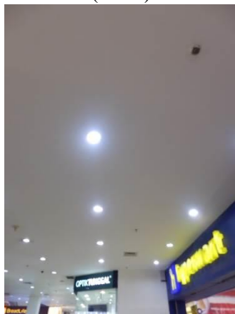
Photos 20: Store passage lighting (Compact fluorescent lamps)
