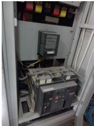
Photo 46: Breaker in the air-cooled chiller distribution board
