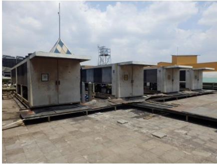
Photo 1: Air-cooled chillers (Mall System 1)
