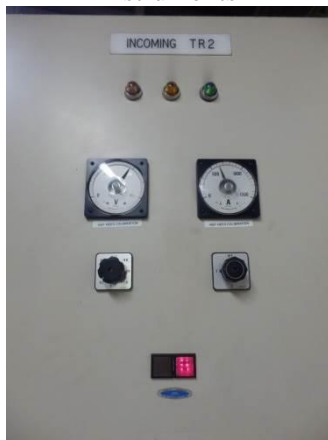
Photo 46: Transformer System No. 2 instruments
