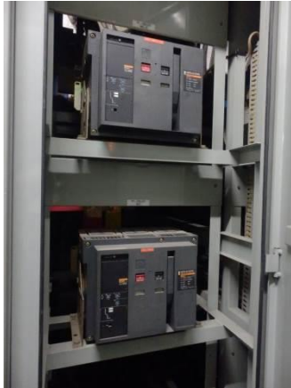
Photo 36: Chiller 2C System breaker (top)
