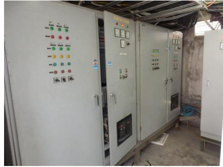
Photo 45: Air-cooled chiller distribution boards (Mall System 2)
