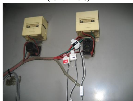
Photo 6: After installation of CT (for lighting)
