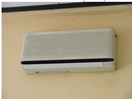
Photo 8: Packaged air conditioning unit (wall-mounted)
