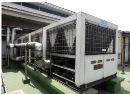
Photo 50: Air-cooled chiller
