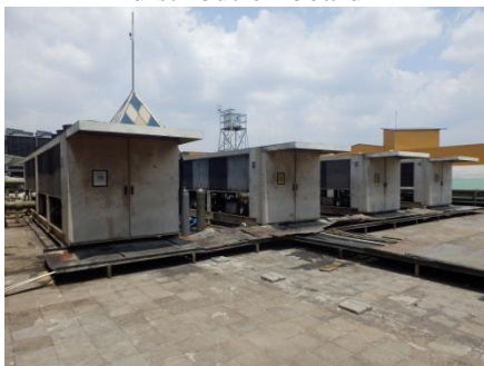
Photo 42: Air-cooled chillers (Mall System 1)
