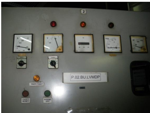
Photo 12: Outside of the low-voltage main switchboard (System A)
