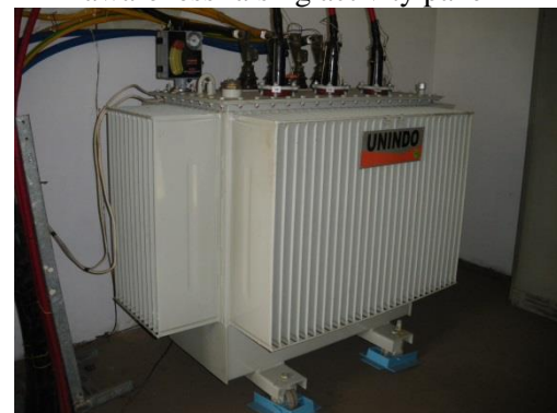
Photo 9: Power-receiving transformer (630 kVA)
