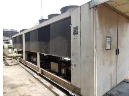
Photo 2: Air-cooled chiller (Mall System 1)
