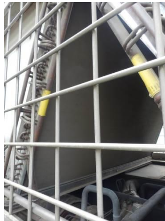
Photo 53: Air-cooled chiller fin tube heat exchangers
