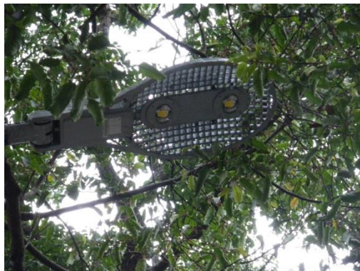
Photo 4: LED street lamp (lighting part)
