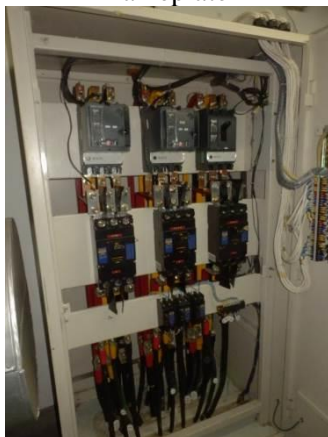
Photo 55: Air-cooled chiller distribution board
