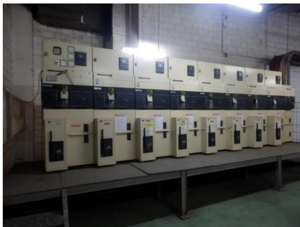
Photo 32: Power-receiving part of the Mall facility
