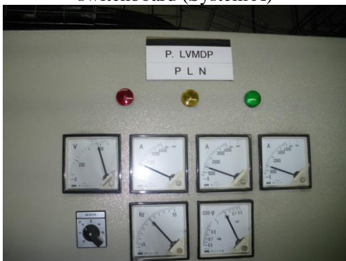
Photo 14: Outside of the low-voltage main switchboard (System B on the 2nd basement floor)
