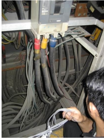
Photo 7: Performing the under-panel wiring work
