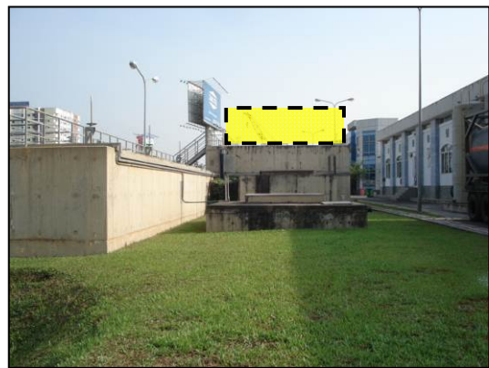
Estimated location to install micro hydropower generator
