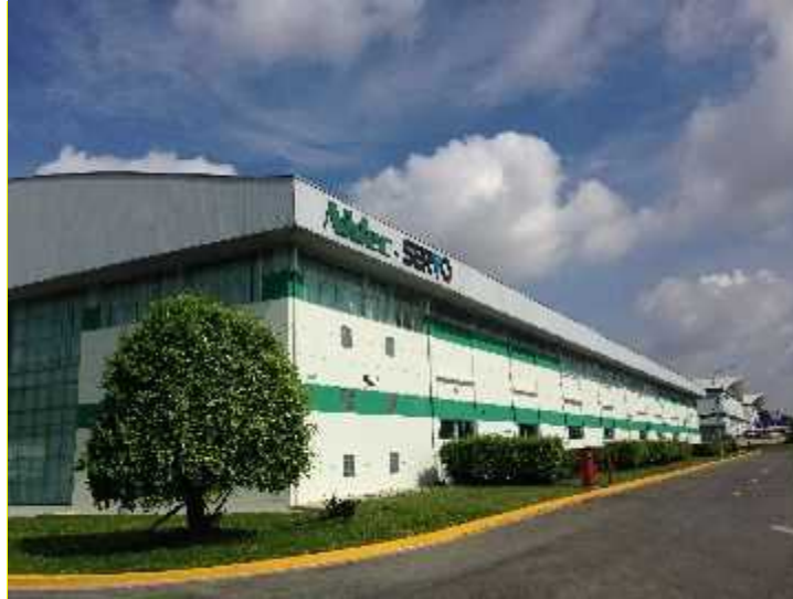
Photo 3.1.1 Nidec SERVO located in Sai Gon High-Tech Park in District 9, Ho Chi Minh City
