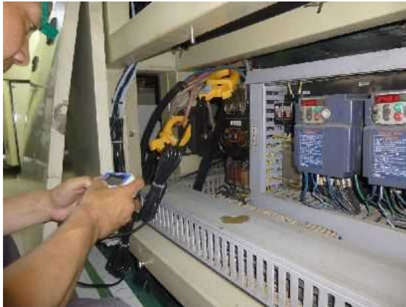
Photo 3.1.6 Checking the pressure of the compressor
