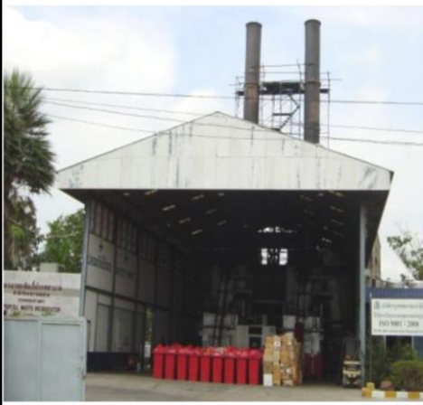
Infectious Waste Incinerator At On-nut Transfer Station Capacity 15 tons /day (x2) Total 30 tons /day
