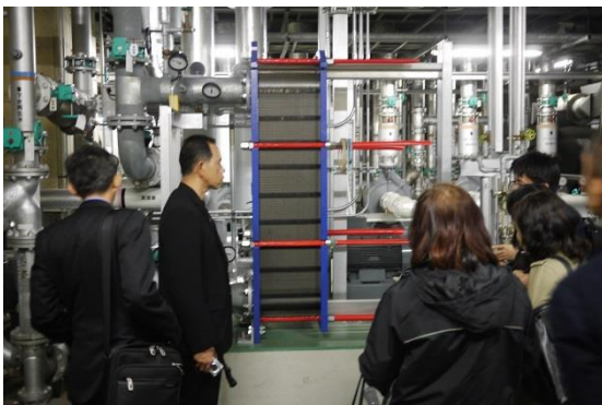
Heat exchanger for wastewater heat
