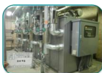
High efficient absorption water cooling heating machine (Top-runner type)
