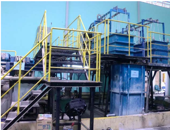
Existing industrial wastewater treatment equipment
