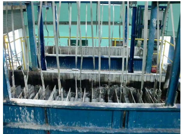
Existing industrial wastewater treatment equipment
