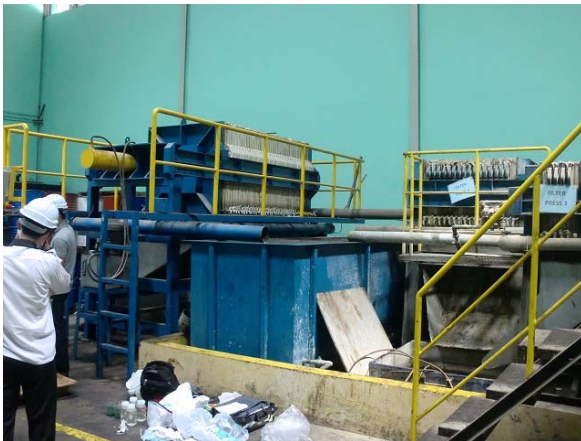
Existing industrial wastewater treatment equipment (belt press)
