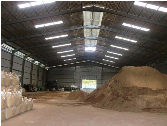
Plant roof (being considered for PV panel installation)
