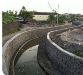
Improvement of urban drainage system by introducing ecodrain concept combining detention (holds water temporarily) with retention (ground absorption)
