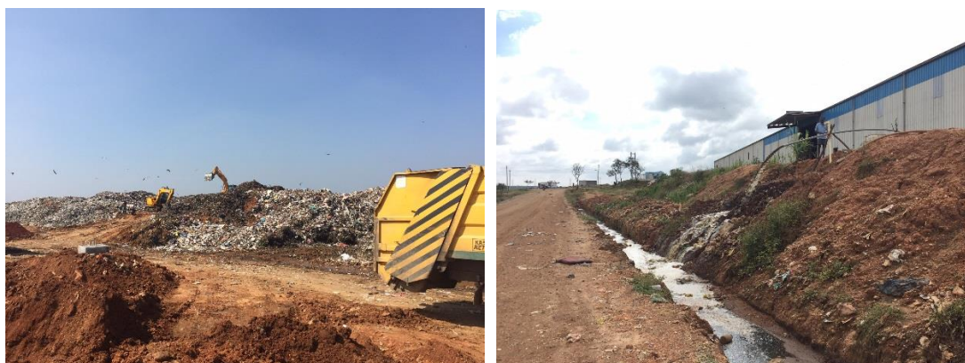
Figure 3-8: Observed Open Dumping in a Composting Facility (Left) and Untreated Leachate Discharged to the Environment (Right)
