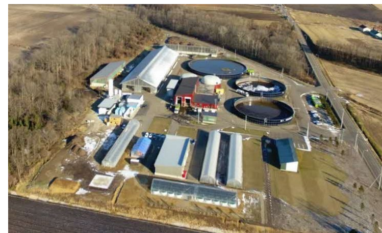
Naka-Shikaoi Biogas Plant (Source: Shikaoi Town)
