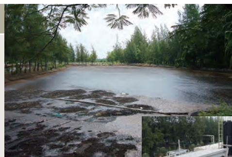
Anaerobic open lagoon
