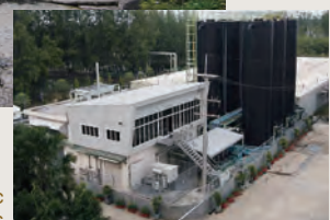
Newly installed anaerobic fermentation tanks
