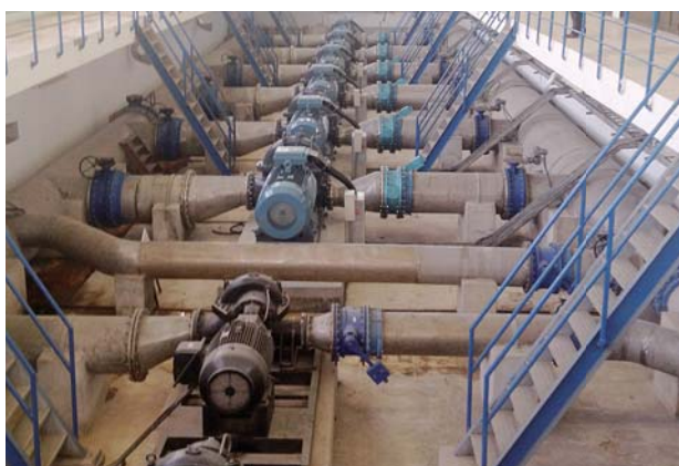
High efficient pumps introduced
