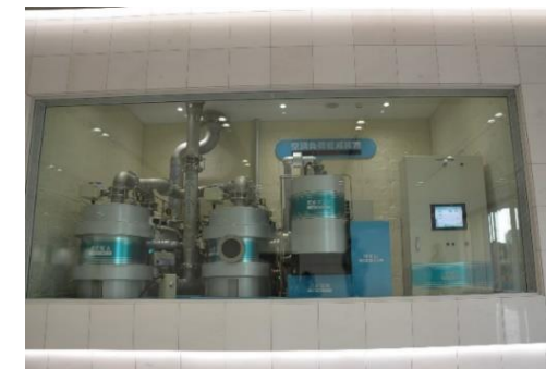
CO 2 capturing equipment for building air conditioning
